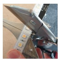
3. Using a pair of scissors cut the strip light to length. Use a single cutting motion in the center of the cut pads.
